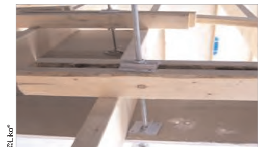
Figure K-11: Threaded Rod Mount
